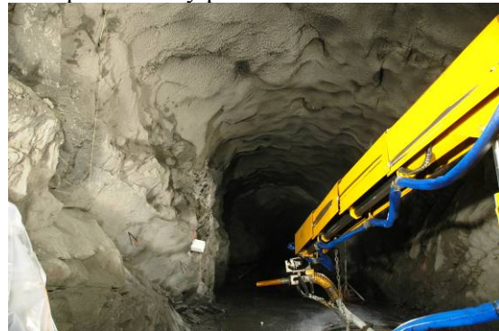
Fig. 3: Horseshoe tunnel profile for the large-scale field test.
