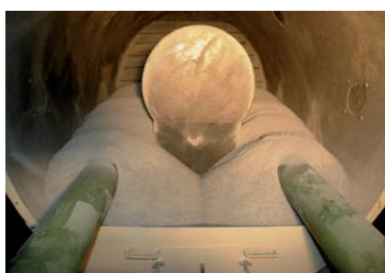
Twin auger system to emplace granular bentonite buffer material around mock-up canister
