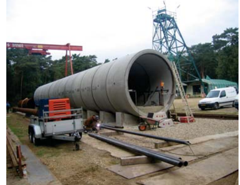
Grout backfill full-scale mockup during construction at Mol
