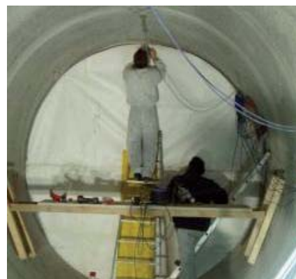
Installation of hydration mat during bentonite buffer construction (2007)
