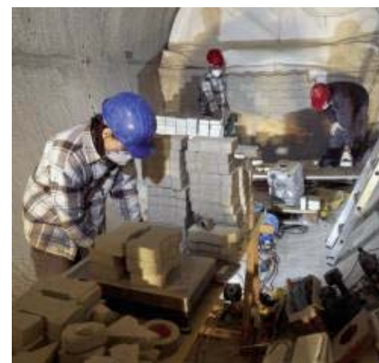
Construction of bentonite block buffer at Grimsel (2007)
