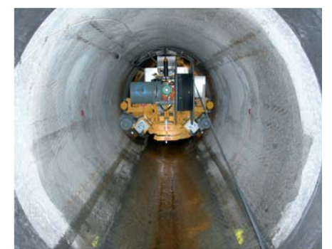
The water cushion deposition machine in the demonstration drift at Äspö
