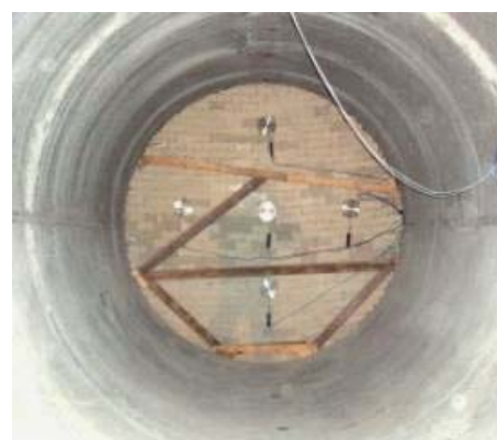
View of bentonite buffer finished
