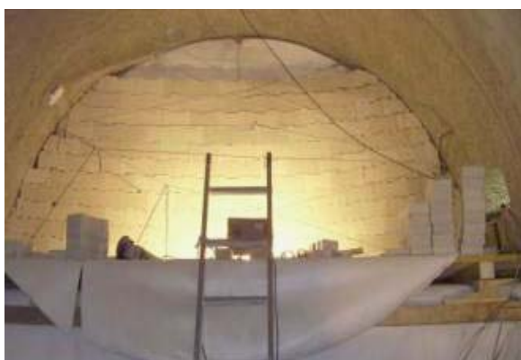
Single bentonite buffer layer almost completed
