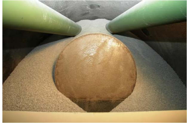
Figure 4: Double Auger (green) Placement of Bentonite Pellets Around a Canister (Nagra)
