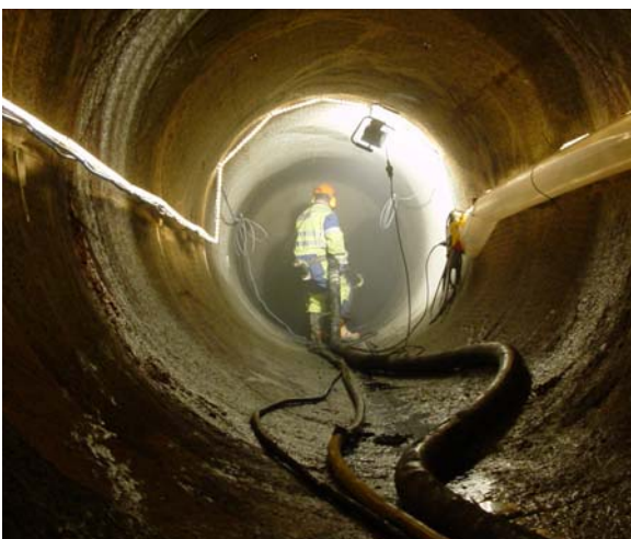
Figure 10: Short Plug Construction at Äspö (Enresa / Aitemin / CSIC)
