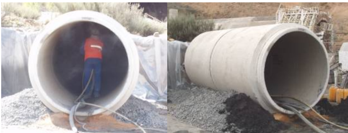
Figure 4: Testing of shotcrete formulation for plug construction in Spain
