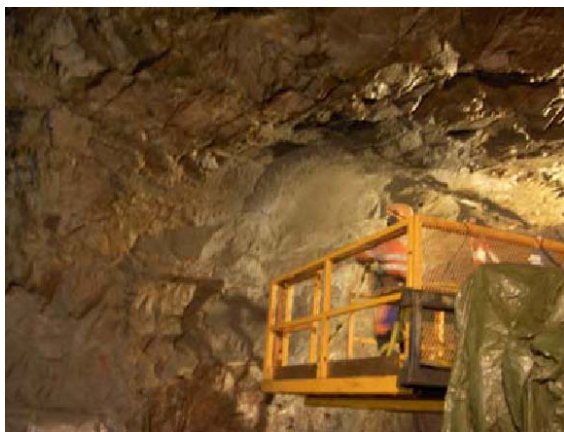
Figure 8: Low-pH shotcrete for rock support: field activities in Sweden (left) and Switzerland (right)
