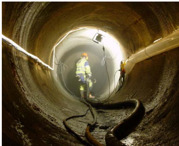
Figure 5: Construction of short low-pH plug in Äspö URL
