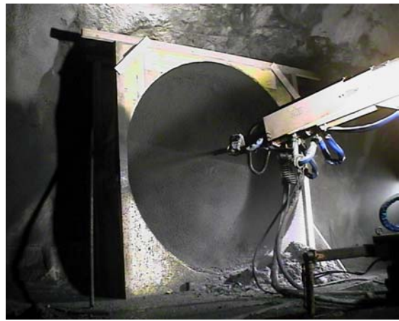
Figure 10: Preliminary shotcreting test in Sargans (Switzerland)
