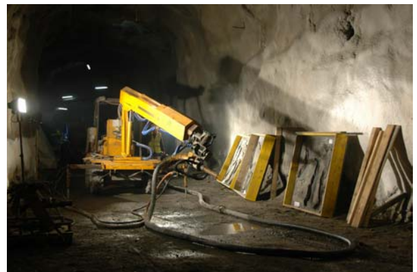
Figure 12: Pilot tests with low-pH for rock support in Hagerbach (Switzerland)
