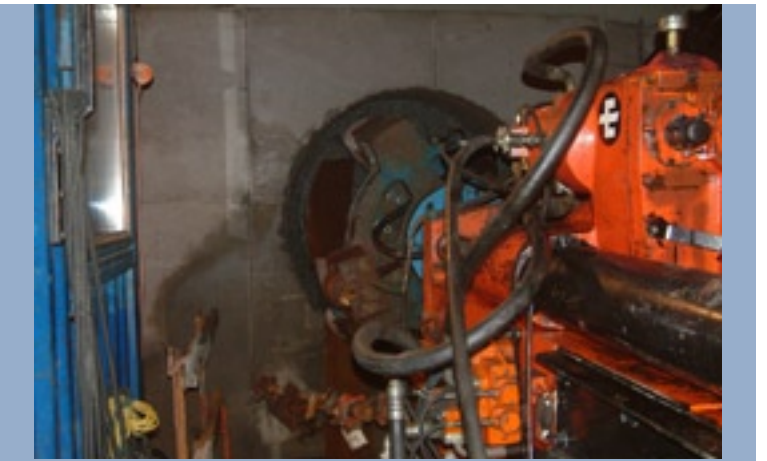
Drilling of deposition drift
