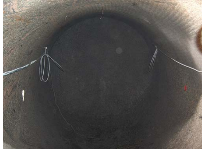
Figure 5: Low pH shotcrete plug constructed at Äspö Sweden November 2005
