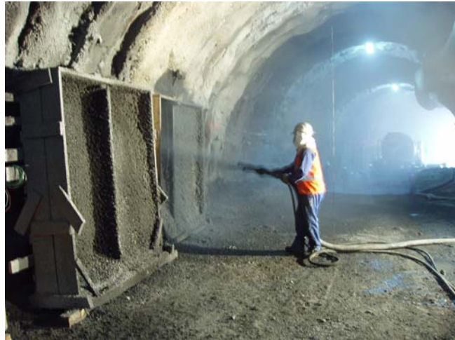
Figure 4: Underground shotcrete test panels at León July 2005
