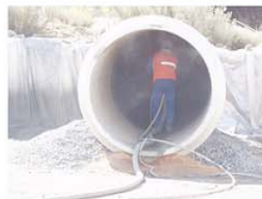
Low pH shotcrete test in concrete pipe León Spain July 2005
