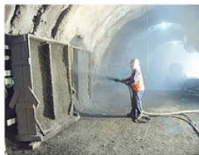
Underground shotcrete test panels at León July 2005
