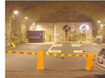
SKB ESDRED underground demonstration room at Äspö Sweden
