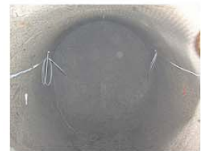
Low pH shotcrete plug constructed at Äspö Sweden November 2005
